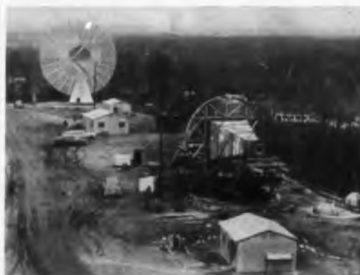
50-ft Horn reflector receiving antenna for Project Echo (foreground) at the Holmdel, N.J., station of the experiment. Other antenna is a 60-ft transmitting dish to bounce 980 mc signals off the satellite to Goldstone, Calif., receiving station.
