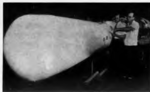
Business end of Project Echo. 100-foot inflatable mylar sphere is packed into nose of Thor-Delta rocket for release 1000 miles up.
