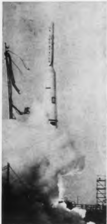
Blasting off into orbit, Pioneer V, packed inside of the third stage of a Thor-Able booster rocket, leaves the pad at Cape Canaveral. The 150-w transmitter carried by the planetoid is about 30 times more powerful than any other previous U. S. space transmitter.
