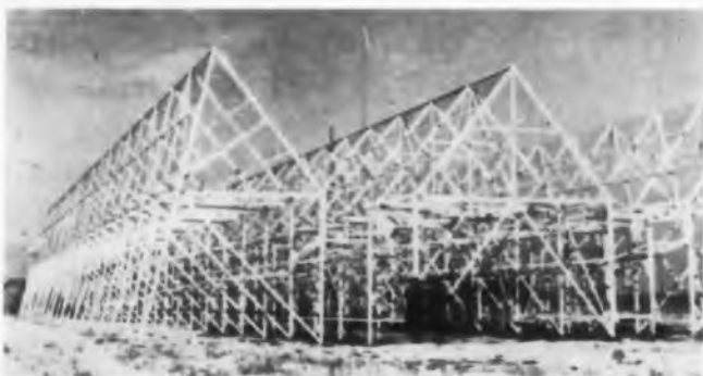
One of the largest corner reflectors ever made is installed at Havana, Ill., to receive radar returns from meteor trails. The 35-foot-high antenna forms a 7-meter double-trough waveguide with an aperture 200 feet long, 70 feet wide.
