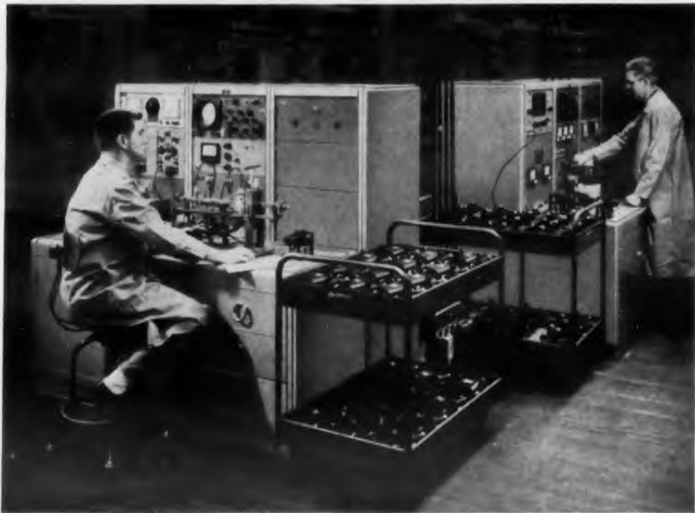
EMCOR Cabinets house equipment for testing of microwave components at the TAPCO GROUP, Division of Thompson Ramo Wooldridge Inc., Cleveland, Ohio.
