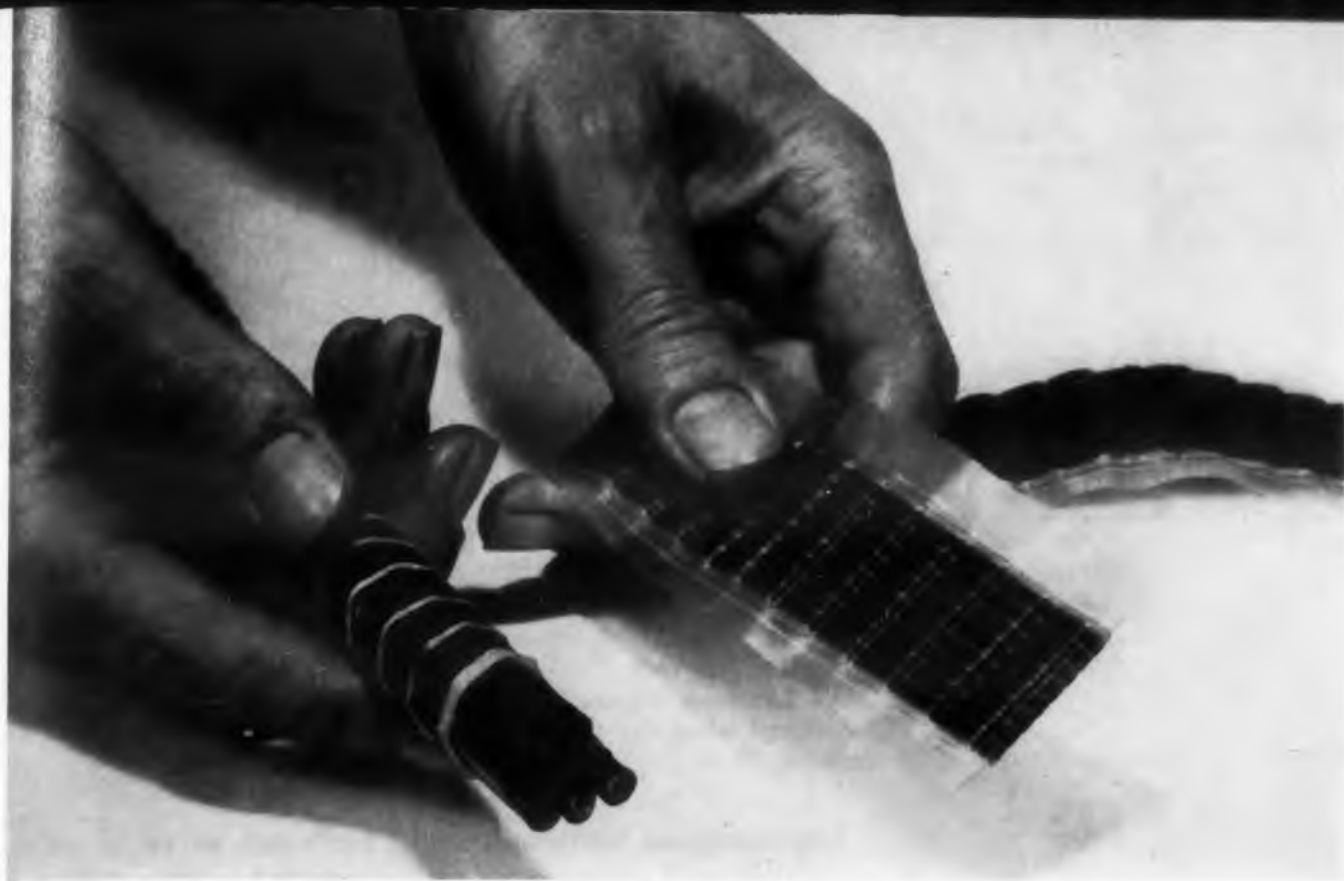
Fig. 2. "Flat-strip" coaxial cable on the right replaces the bundle of coaxial lines on the left.
