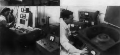
**VIBRATION TEST** checks units from 5 cps to 3,500 cps up to 50 G's. This test normally is performed with direction of vibration applied through each of three mutually perpendicular axes. ELECTRICAL TESTS fall into many categories. These are typical: measuring coil resistance, testing pickup and dropout current, checking dielectric characteristics, and testing millivolt drop across contacts.
