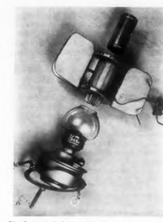
Fig. 2. Method of assembling the lamp and the generator
