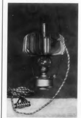
Fig. 1. Thermoelectric generator installed on a lamp, with the connecting plug to a radio receiver.
