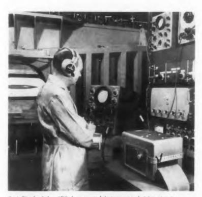
2. 1. Woodard, Jr., ARO. Incorporated, instrument technician, operates the Visicorder in the measurement of aerodynamic damping coefficients.
