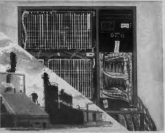
PROCESS CONTROL EQUIPMENT—Process controls, instrumentation, and other industrial electronic equipment can be more reliable and more easily serviced at reduced costs with TFE resins. They have zero moisture absorption, are non-flammable, and are chemically inert. Neither potting temperatures nor soldering iron heat will damage TFE resins.
