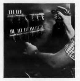
Colloidal graphite is spray-applied on grid plates to increase radiation, reduce secondary emission.
