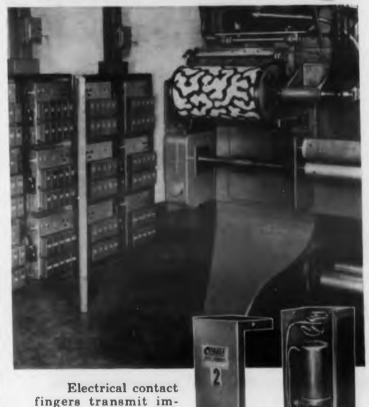
Electrical contact fingers transmit impulses to 120 CLARE RELAYS each housed in a modular type unit.
