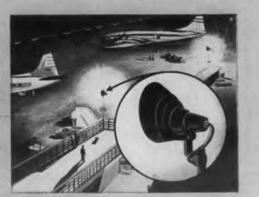
SPECIALTY FIXTURE WIRING -Non-flammability, resistance to heat, moisture and aging of TFE resins assure reliable performance of floodlights, heat lamps lighting
