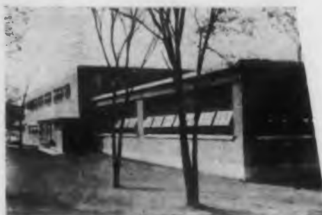
▲ Plant of Westchester manufacturing subsidiary, Pleasantville Instrument Corporation; additions are under construction.
