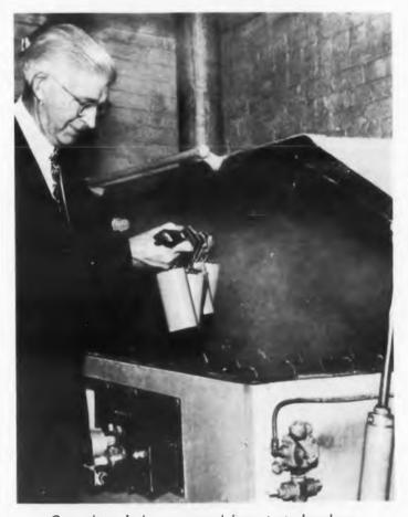
Capacitors being removed from test chambers.
