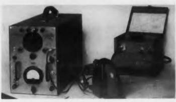
This 35 lb portable magnetron tester, Type 162, will qualify magnetrons in the field, making it of value to users of all types of radar equipment. It will evaluate a large number of magnetron types in present manufacture and use. The main indicator unit is supplied from 115v 60cy and requires approximately 150w.
