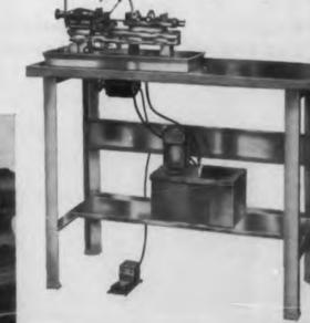
The cross slide has a swivel slide at one end and a rigid tool block at the other. Lever collet closer provides quick opening and closing. A variety of turret tools with 1/2" shanks is available.
