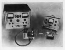
A complete line of 5mm equipment, operating over the full waveguide frequency range of the RG-98/U waveguide (50.00-75.-00kMc), has been made available by this firm. A slotted
