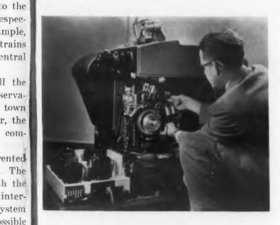
The working parts of an electronically controlled camera that helps prepare directories.
