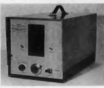
The Type 33-110 "Sadie" Digital Voltmeter has a sensitivity such that 100mv provides full - scale digital output (999). Controls permit selection of any voltage in either of two ranges
