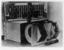
The Model 2E-408 Cabinet Cooling Fan is specially designed to fit the standard 19" electronic rack. It pressurizes the cabinet with filtered air, preventing dust from entering
