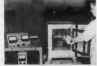
Relays operating in special constructed ovens are subject to temperatures exceeding 400° Fahrenheit. Recording instruments indicate any malfunction.
