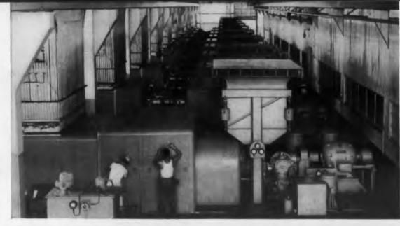
PROCESS CONTROL—Askania controls regulate speed of the ten turbines which develop compression to maintain gas suction pressure in Creole Petroleum Corporation's giant, pile-supported oil drilling operation on Lake Maracaibo, Venezuela.
