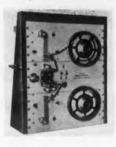
With start and stop times of 5millisec and tape speeds up to 60 ips, the Model 903 Perforated Tape Handler offers character readout of 150, 300, or 600 per sec. It will actually
