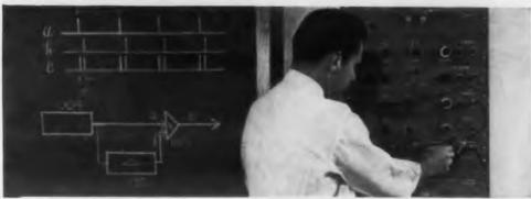
**FAST SET-UP.** Engineer draws pulse sequence, then determines by block diagram how to connect his Burroughs Pulse Units. Usually this can be done in a matter of minutes.
