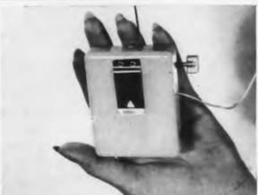
The back of the radio showing the pocket clip. The tuning knob is turned out for the 110Mc signal.
