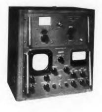
The FXR Spectrum Analyzer, designed for greater accuracy and convenience in microwave spectrum analyses, provides push-pull deflection to both the horizontal and vertical plates. Versatility of the
