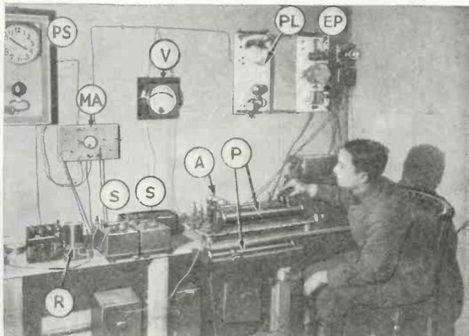
The above photograph shows the installation. PS is a synchronized pendulum, MA is a milliammeter, V a voltmeter indicating the voltage passing through the photo-electric cell, R is a relay, A shows a bank of three amplifying tubes, P shows the potentiometers, PL the free pendulum, and EP the photo-electric equipment.
