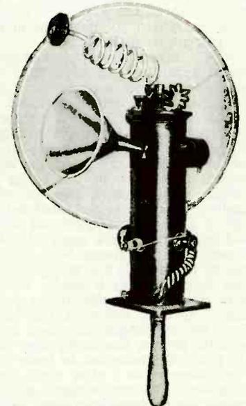
This particular device is made of a metallic tube, approximately 12 inches long. A funnel is soldered to the can and projecting from the top is a coiled aluminum tube, attached to a metal disk. There is a rheostat in one side and a switch at the back, purely for impression. The cap is exploded by action of the thumb or finger.
