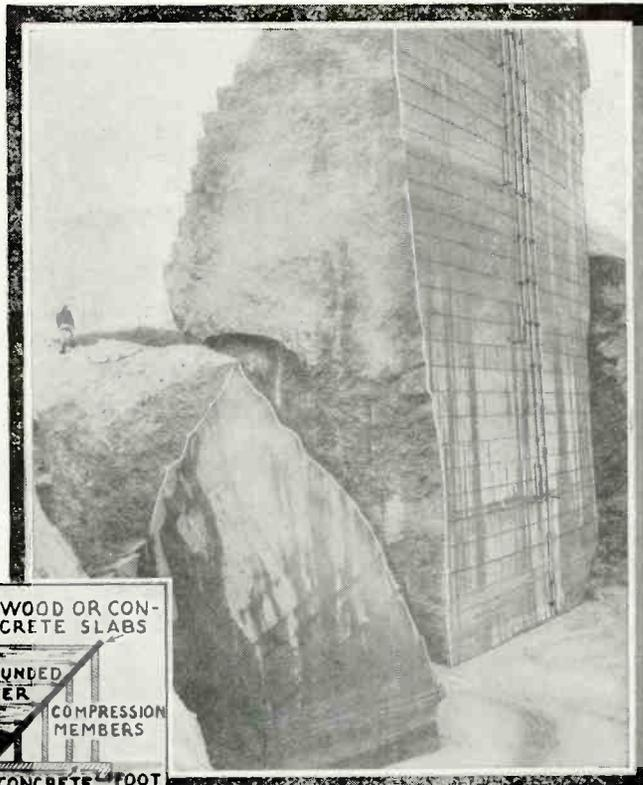
The St. Francis Dam was of the gravity-arch type illustrated. An odd type of dam is the wedge shape design illustrated. The method of dividing large concrete dams into several sections to allow for expansion, is illustrated.
