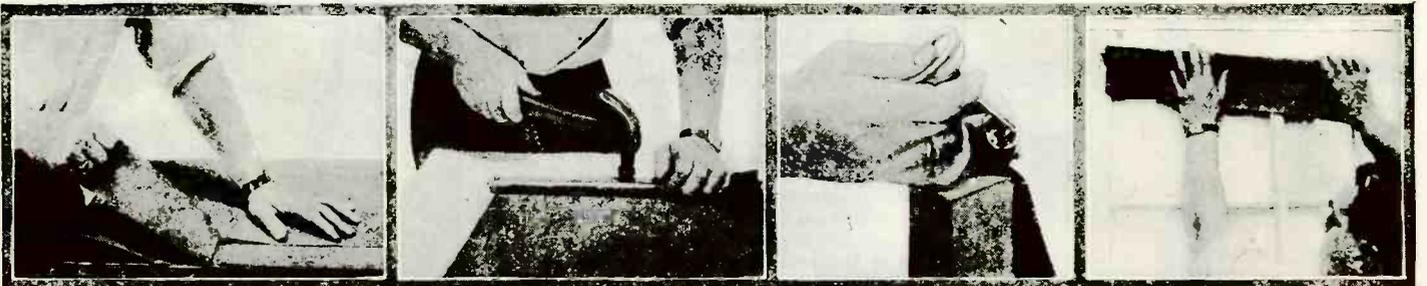
Above—tearing the cloth to size. Tacking the cloth on the roller. Oiling the trigger for free movement. Fitting finished shade in place.
