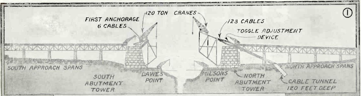
The illustration appearing above shows the first stage in the construction of the single span bridge. Both sides of the harbor, with approaches and abutment towers, are shown. The creeper cranes weigh 570 tons each and will lift 120 tons. The anchorage cables are only temporary.
