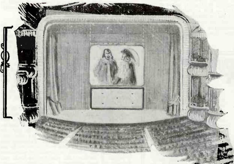
At the left is an illustration showing how the huge cone speaker is placed in back of the screen at the bottom. This in no way interferes with the picture and when the screen is raised the loud speaker clears the proscenium arch.
