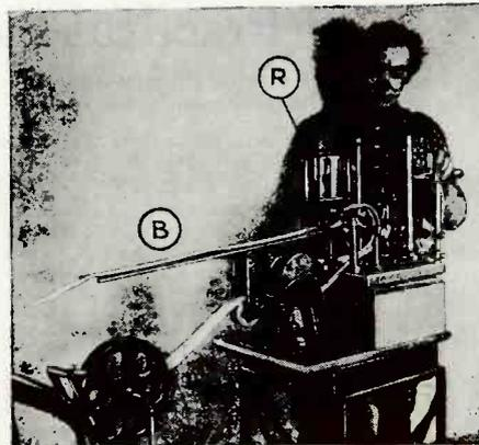
The above photograph shows, at B, the paper strip, and the water reservoir at R.
