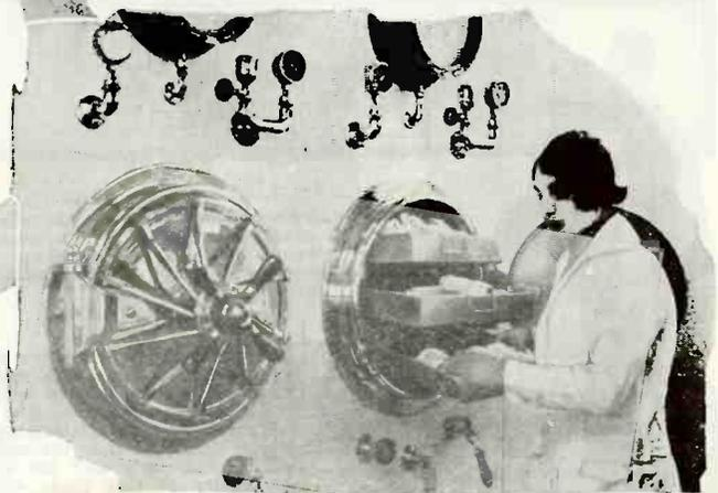
New cabinets for the sterilization of dental and surgical instruments employ super-heated steam. The above is installed at the New York University College of Dentistry, and is demonstrated by Miss Kathryn Blond.
