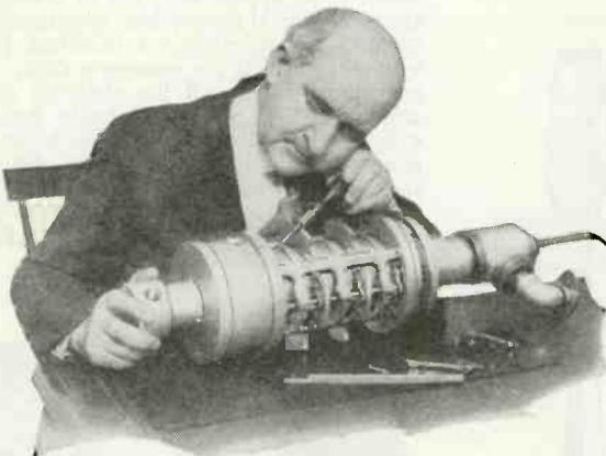
An airplane motor which weighs but fifty pounds is shown above. With the exception of the ball bearings and adjusting screws, the motor has but four major parts and has no valves or springs. The single cylinder acts as a cam to separate the intake and exhaust. The inventor, Edwin L. Rice, claims that the motor is equivalent in horse power to a 450 pound motor. The motor is capable of making 200 miles per hour.
