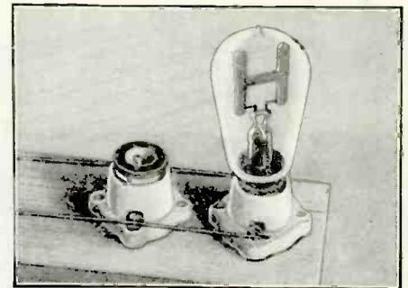
When the fuse shown here blows, the neon lamp lights, indicating the fact.
