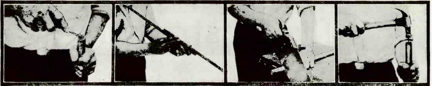
Prying off metal tip before cutting roller. Two sticks can be used to measure width of window. Cutting the roller to fit the window. Driving the tip into end of roller.
