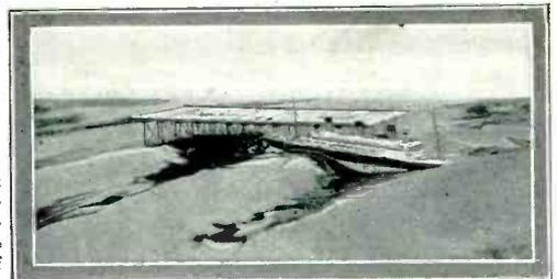
Photo at right shows model of seadrome and also model of steamship "Majestic" under test in tank with 50 to 60 ft. waves; note that platform is practically level, while steamship "Majestic" is diving downward, practically overcome by the huge waves. The average height of ocean waves is 50 ft.
