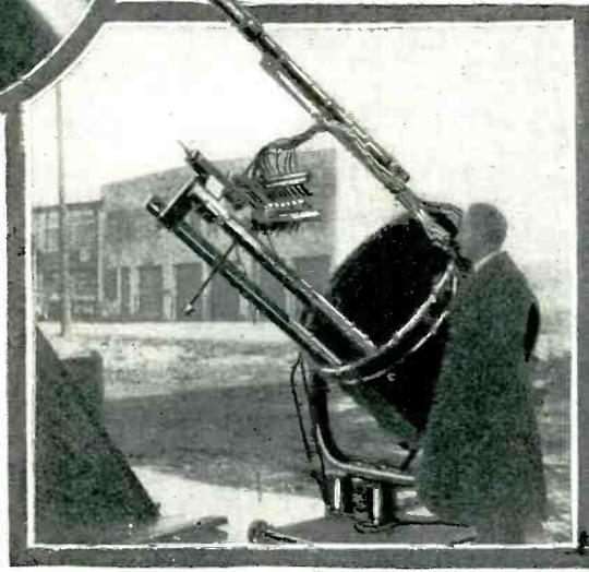
Photo above shows construction of projectograph arc light. The horizontal carbon made in the shape of the letter to be cast, may be seen at the end of the two focusing rods. A mechanism is provided which permits the horizontal carbon to be adjusted and removed for replacement. The reflector is rather flat, so that the light may be concentrated at a distance, and the distance of the arc from it is easily adjustable.
