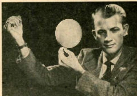
**SOUND WAVES** that are passed through a lens-shaped area of a gas that is heavier than air will come to a focus much the same as light waves passing through a glass lens. You can demonstrate this with the balloon that was filled with carbon dioxide gas in an accompanying experiment. Hold the balloon between your ear and a ticking watch. By maneuvering the balloon you will find a spot in which the ticks sound considerably louder than they do when the balloon is removed.
