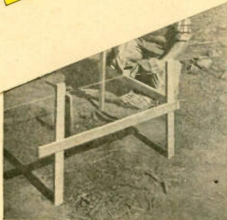
When batter boards are being placed for a second corner and the established line does not reach, extend the line over the second measured stake, as above. Shift the line to align with a saw kerf in the stake and mark it on the batter board.
