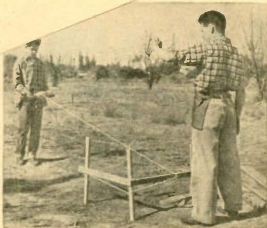
Approximate squaring of a line to locate a far corner is done by sighting on a framing square lying on the ground. Below, a screed cleated to slide on the side of the form reveals uneven spots on the base surface.
