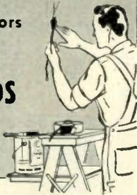
The soft, non-hardening plastic material of Press-Tite Caulking and Sealing Cords is the quickest, easiest and neatest method of filling unsightly cracks and holes in wood or plaster before painting.
