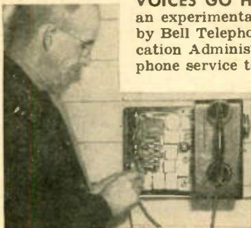
Mrs. Carl Robbins puts through one of the first calls to go over the new power-line phones, while William Hickox, left, completes an installation. The equipment in the box produces a high-frequency carrier current.
