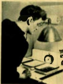
A No. 212 enlarger lamp 2' away gives the second exposure. Examine print through filters to find which to use.
