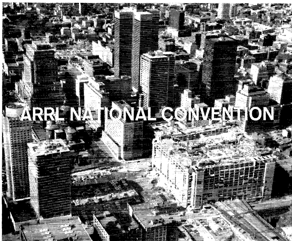
Place Bonaventure, with its penthouse hotel, under construction in downtown Montreal.
