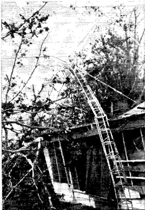
This is the result of Typhoon Sally on the beam at KG6CK. See the Diary for further details.
