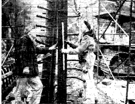
W1QZ and W1QXX lining up the mount for new dish at W18U.
