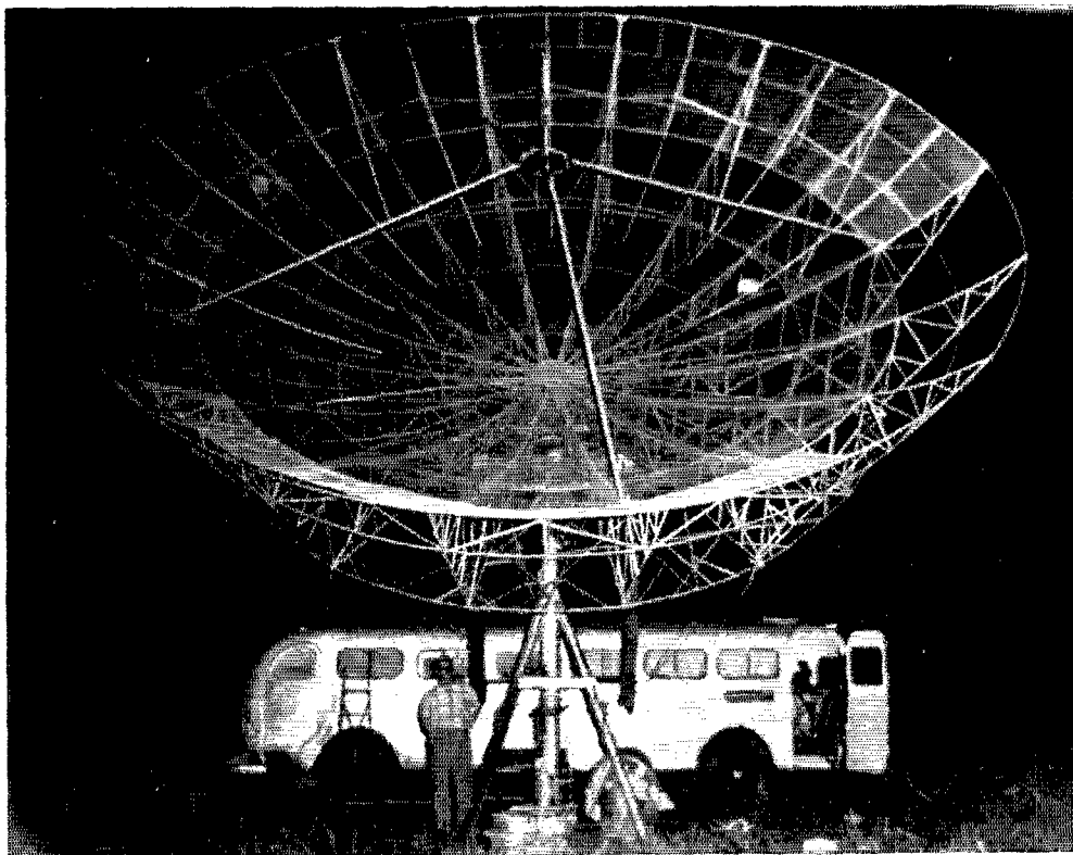
W8LJO's almost-completed 26-footer for 1296 Mc.
