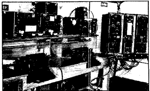
Station of Naval Reserve Electronics Platoon 6-23, Belle Glade, Fla. This station has been of considerable assistance in hurricane emergencies during the past four years.
