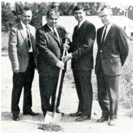
John and Dan Mezzalingua break ground for an addition to the manufacturing plant. Looking on (l to r) are Joe Gibbs and Keith Morgan.
