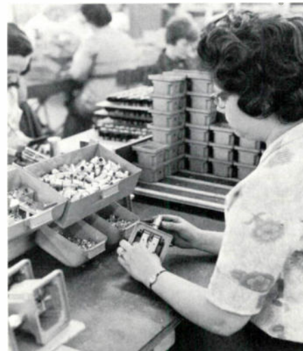
Modular directional tap assembly station.
