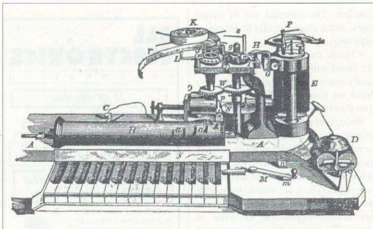
**Photo B.** 1860s printing telegraph. The "piano keys" are linked to the characters of the alphabet.
