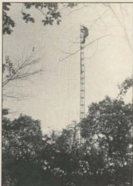
Photo B. Dave Porter K2BPP atop the 40-ft level, getting ready to put up the last 10-ft tower section.
