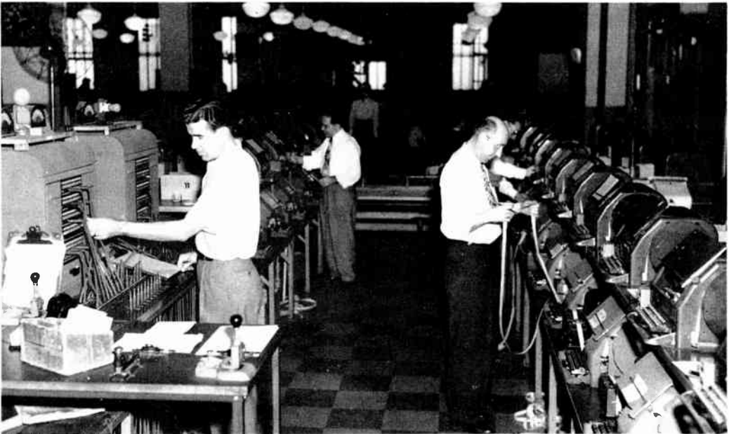
Receiving and sending equipment in the New York switching section
