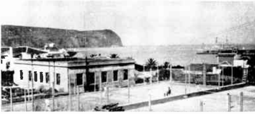
Power house and harborside locality below operations buildings. Across the bay, the precipitous cliffs are typical of the island seacoast.
