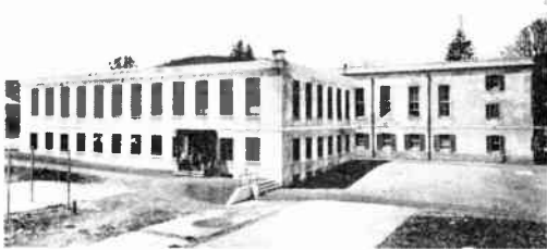
Operations buildings at Horta as they appeared early in 1928 shortly after completion of the new structure in foreground.
