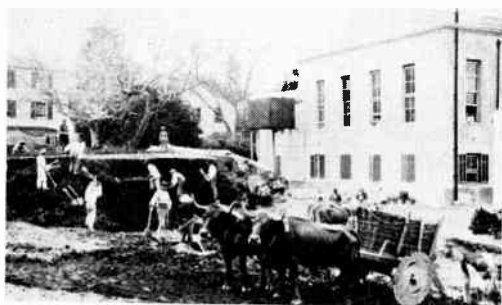
Wooden wheeled ox-carts like large basket-weave chariots moved many tons of rocks, earth and building materials for the Horta station.
