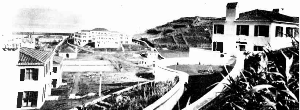
Residences of Western Union Director (right), Superintendent and Chief Electrician (left), recreation building (beside tennis courts), and two-family dwellings and staff house (center).
