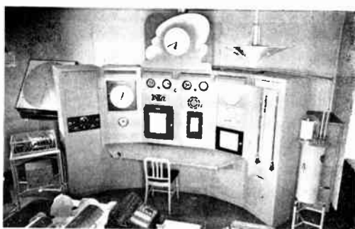
Instrument racks in Weather Bureau office, Washington, D. C.
