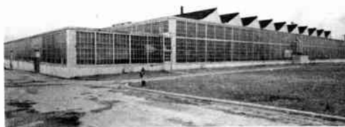
Figure 1. Main shop building — Chattanooga Works
