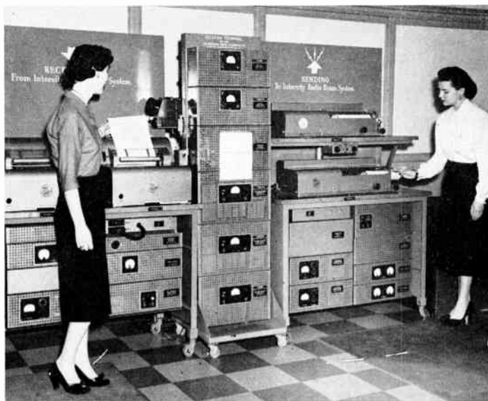
Figure 1. A complete High-Speed Facsimile terminal
