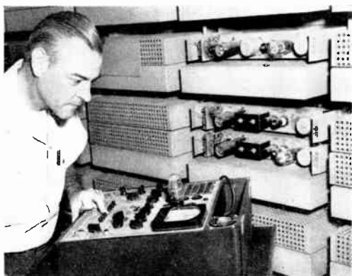
Service interruptions can often be forestalled by the periodic testing of vacuum tubes
