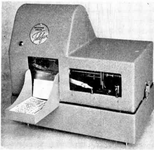
Message-a-minute facsimile telegram recorder used in mobile Telecar motor delivery service
