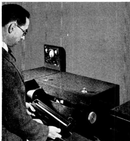
Cablephoto film recorder was designed for Western Union's transatlantic picture service
