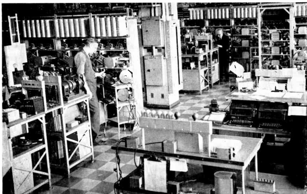
Figure 2. Varioplex Central Office equipment.
