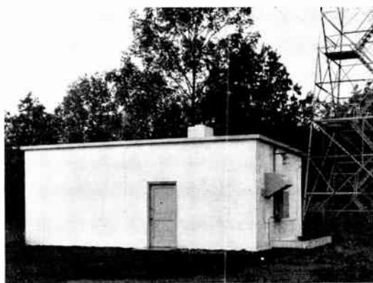
Figure 9. Typical equipment building at relay stations, housing the rack equipment and power plant
