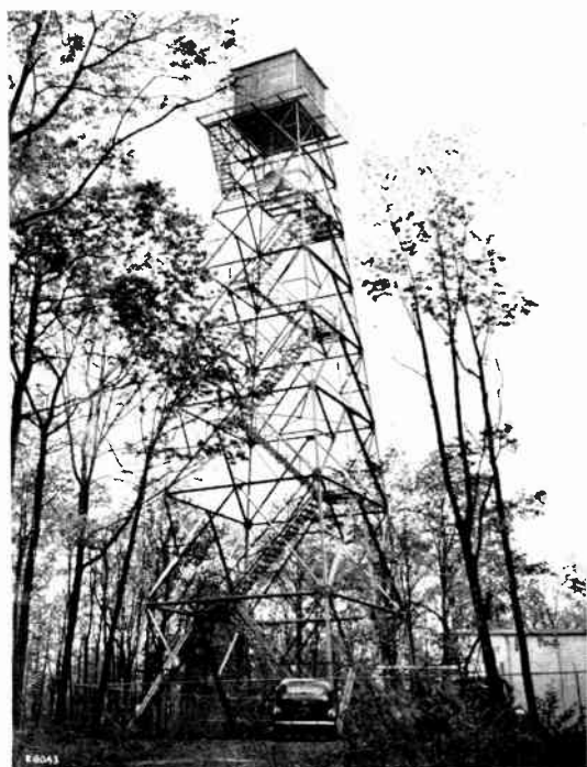
Figure 8. Typical relay tower on the New York - Pittsburgh - Washington triangle. The transmitting and main receiving antennas are in the tower cabin behind the fibre glass windows; the diversity antenna is about twenty-five feet below
