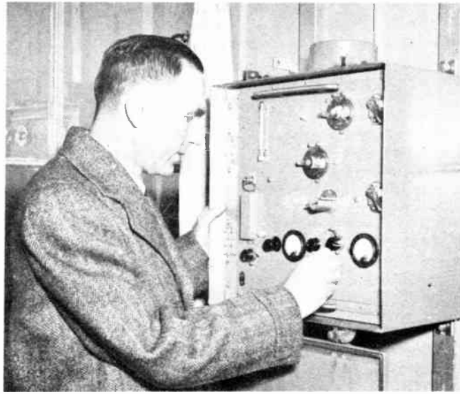
Weatherproof Microwave Equipment Cabinet Used for Remote Amplifiers.
