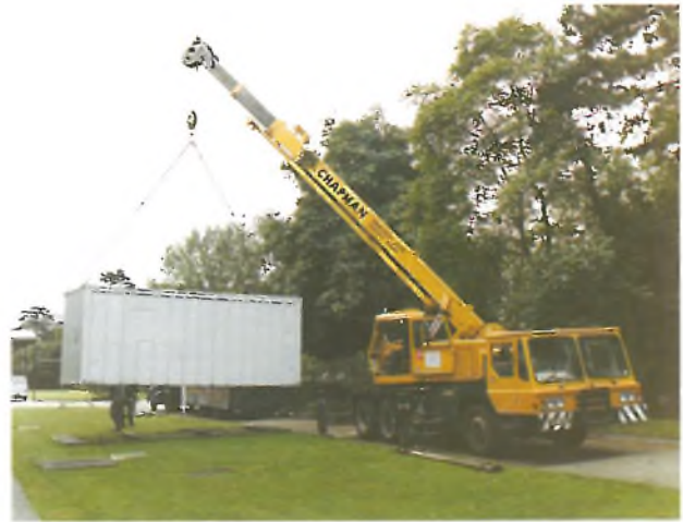
Fig. 5. Loading the mobile laboratory on to a transporter.
