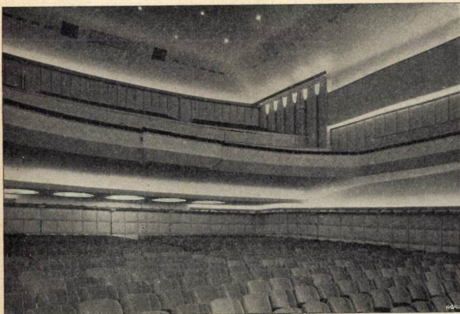
Fig. 6. View from the stage into the auditorium. Attention is called here to the form of the ceiling under the balcony which gives the appearance of a thin free-hanging shell in which circular holes are pierced and above which the upward sloping, brightly lighted ceiling of the balcony is suspended. In the ceiling of the auditorium may be seen the regularly spaced small holes through which direct light is thrown upon the audience.
