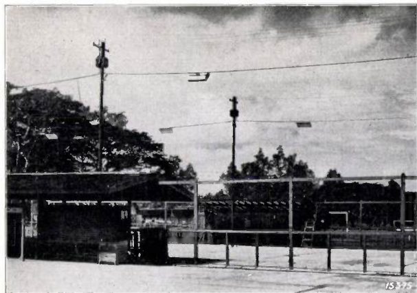
Fig. 1. Lighting fixtures of tennis courts with sodium lamps illuminated.
