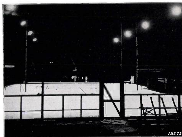
Fig. 2. Tennis court with sodium illumination.
