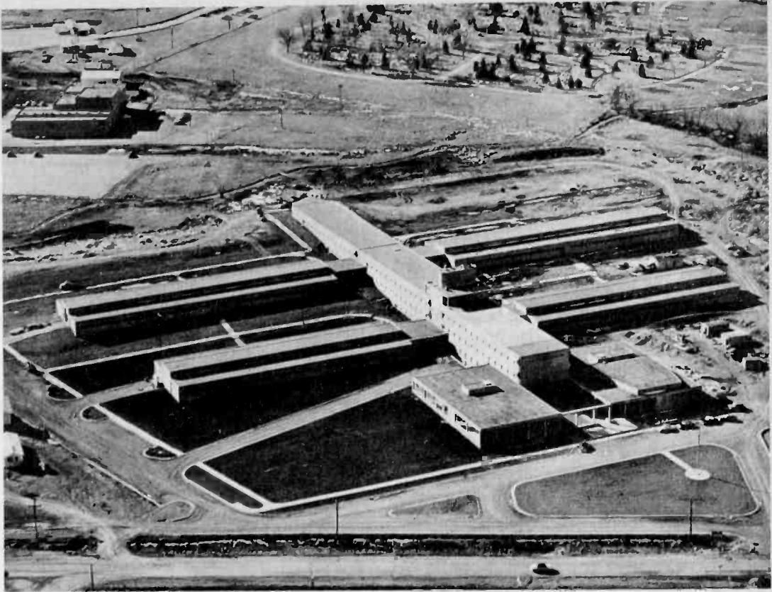
Figure 1. Air View of the National Bureau of Standards Multimillion Dollar Research Center in Boulder, Colorado. This structure will house the Bureau's Central Radio Propagation Laboratory. The design of the building features a central spine, with one-story wings extending perpendicularly from it on either side. The structure takes advantage of the sloping terrain that rises from a state highway toward the Flatirons to the west. The buildings in the background, also part of the research center, are portions of the NBS-AEC Cryogenics Engineering Laboratory.
