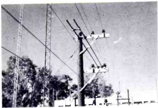
Filtering Coplanar Mounted Upon a Support Pole
