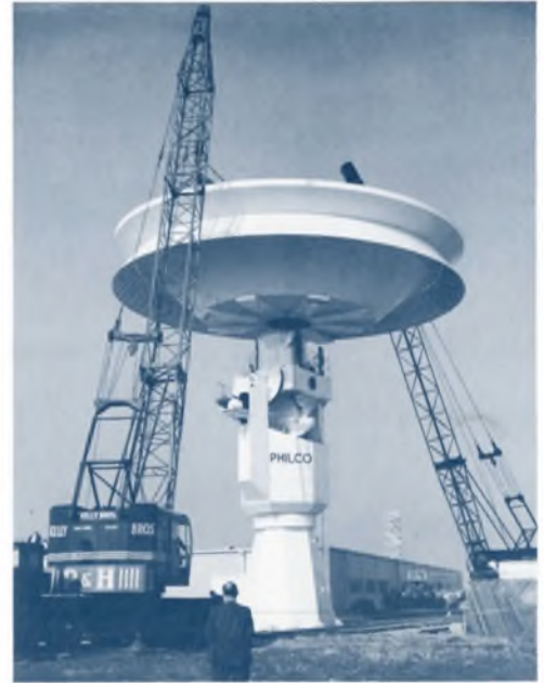
The Philco Big Dish Antenna, now installed at the Vandenberg Air Force Base, where it is used for trailing satellites such as the Discoverer and Midas.
