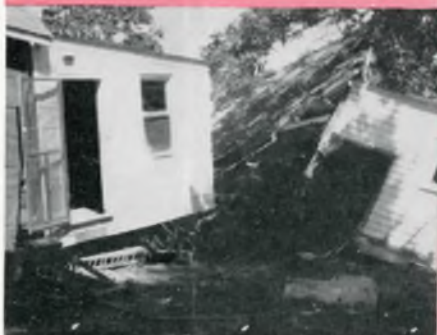
◀ HOUSES ON RIVERSIDE ROAD in the Fergusonville area damaged by the flood.
