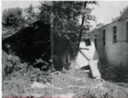
◀ THESE TWO HOUSES in the Fergusonville area were a total loss after flood waters removed them from their foundations and struck them against a solid masonry constructed house.
