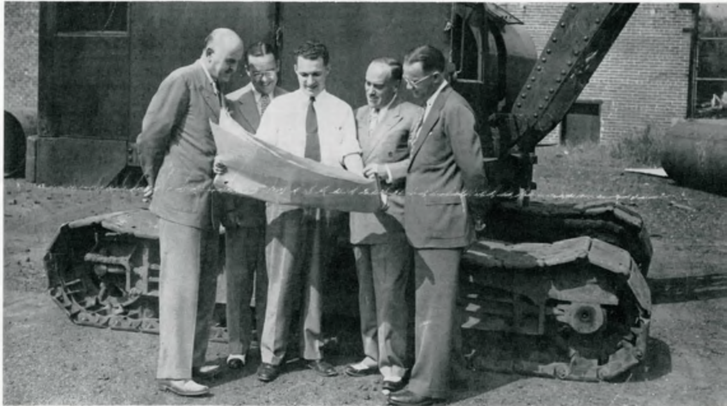
Philco officials look over plans for the new radio-phonograph plant just before excavation starts. Left to right: William Balderston, vice-president in charge of operations; William Peltz, general production manager; H. N. Johnston, manager of the maintenance
