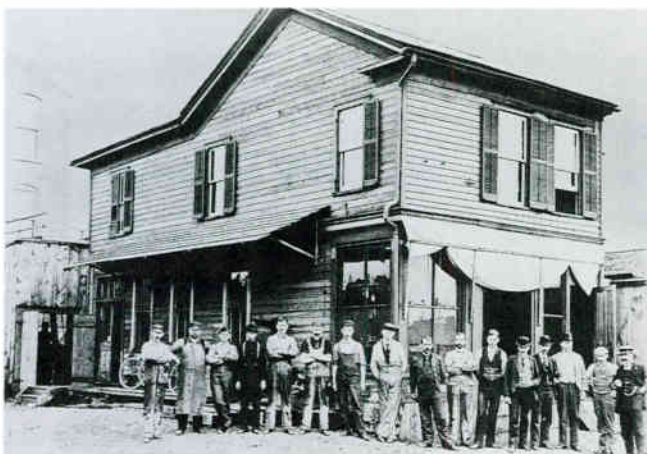
The company's first plant was two rooms in the house at Niles, Ohio where U.S. President William McKinley was born
