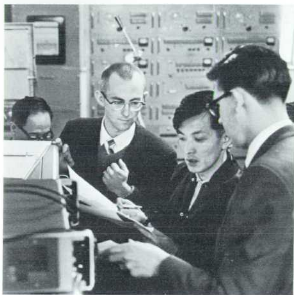
Fig. 3. Operation of traveling cesium-beam clock is checked by -hp- Engineer Richard Baugh before start of ocean-spanning journey. Cesium-Beam Frequency Standard (middle instrument) has self-checking feature that enables adjustment of cesium-beam resonator for correct operation without reference to any other frequency standard.
