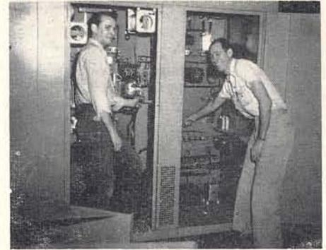
Jim Gibson and George Van De Boe are completing the final assembly of a BC1-F. Here the complete installation of all sub-assembly work as well as additional miscellaneous parts can be seen.
