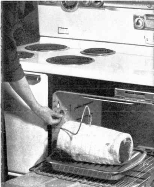
A GLANCE AT THE DIAL on the back panel of the 1956 range reveals the internal temperature of the roast in the oven . . . an electric thermometer does it. At right above, the new speed griddle.
