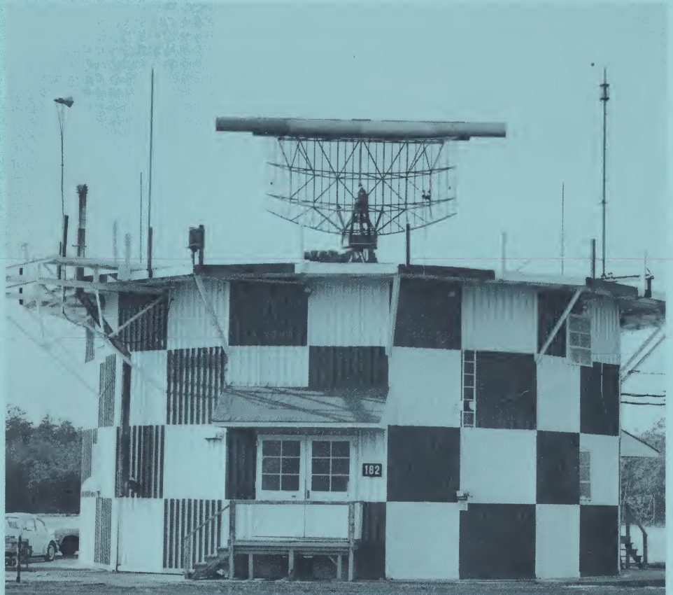
General view of FAA's Terminal Radar System, Model ASR-5.
