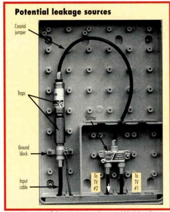
Potential sources of signal leakage at the ground block location
