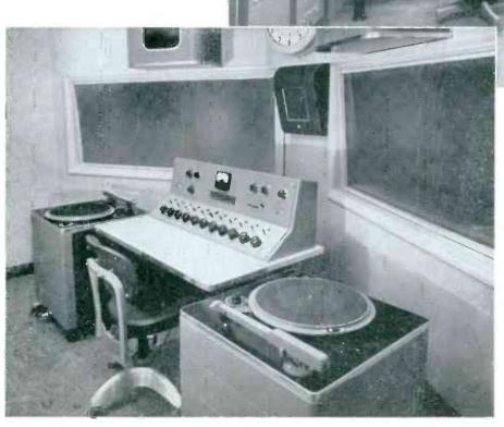
WJPG-FM, Green Bay. One of the specially-built studio-control consoles in WJPG-FM's 4-studio arrangement. Complete two-channel operation (AM and FM), simultaneous audition and broadcast from any combination of studios. remote lines, cueing and talkback are provided.
