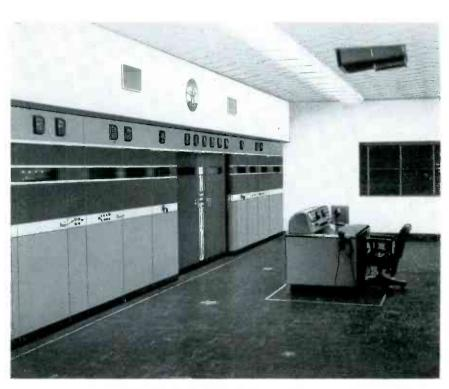
and may be located in the transformer vault or at the rear of the transmitter. A typical transmitter installation requires a space of only 33 x 17 feet for transmitter and associated control and power equipment. A control console finished in umber gray to blend with the transmitter styling is furnished.
