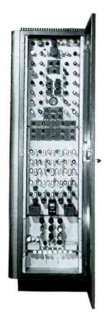
the back of the panels, and are accessible through the rear door. All terminals are in the clear, and components are identified so that circuit testing, when required, is relatively easy.
