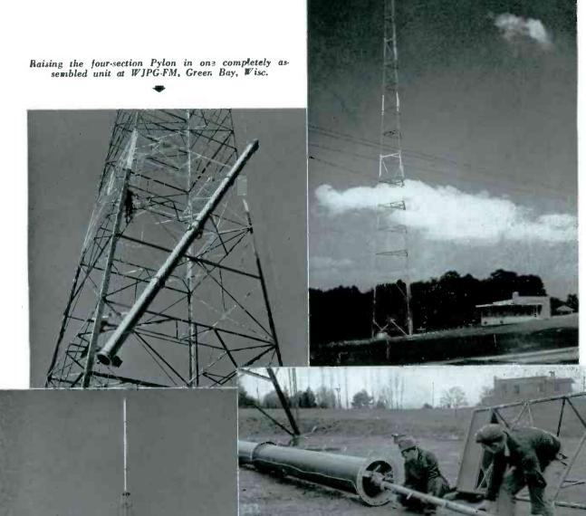
Inserting the transmission line harness into the two-section Pylon at WSBA-FM, York, Pa.
