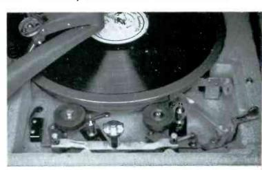
OFF-78 RPM—In the "OFF" position a brake shoe is applied to the turntable rim, and rubber idlers are moved away from both the drive whee and turntable rim.
