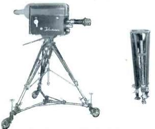
TD-11A Tripod above with RCA Studio Camera. At right TD-11A is collapsed for carrying.
