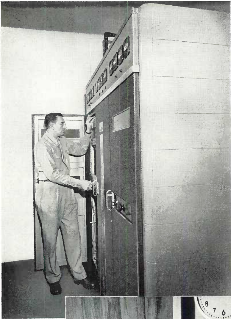
◆ Making adjustments on the three kilowatt FM transmitter, Type BTF-3B, at KSCJ-FM, Sioux City, Iowa.
