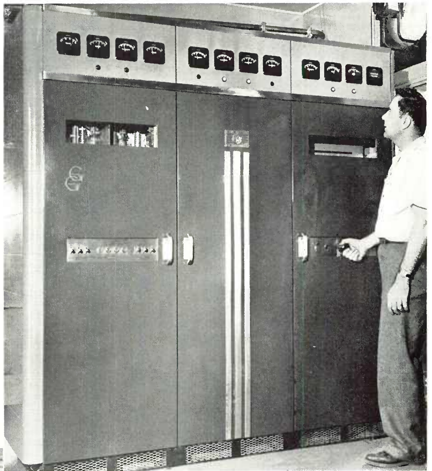
Adjusting line voltage on the three kilowatt FM transmitter, Type BTF-3B, at WGP4-FM, Bethlehem, Pa.
