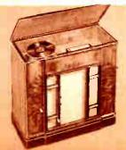
MODEL PE-146 Automatic Combination (Illustrated above). This splendid cabinet houses lustrated above). This splendid cobinet houses both the Lafayette II-tube 5-band Superhet and the Standard automatic mixer-changer that plays 12-10" or 10-12" records automatically. Hi-Fidelity crystal pickup. Overall cobnet dimensions 33%" high, 16" deep and 34%" wide. For 110-120 V. 60 cycles a.c. operation. Complete with tubes. Shpg. wt. 135 lbs.
