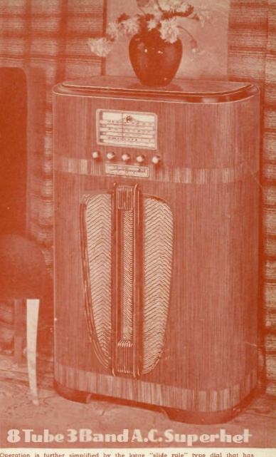
Operation is further simplified by the large "slide rule" type dial that has each band individually calibrated, and the cathode ray tuning "eye" that insures hairline accuracy at all times.
